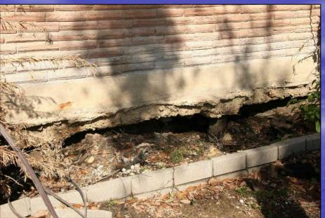
Most residential structures in New Orleans are founded on wood pilings 6 to 8 inches in diameter, driven 30 feet deep. The ground beneath these post-1950 homes has settled 10 to 18 inches.
